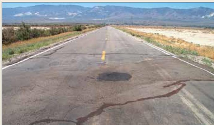
Repairs to State Route 247 after fissures near Lucerne Lake damaged the road surface. Photograph by Michelle Sneed, U.S. Geological Survey.
